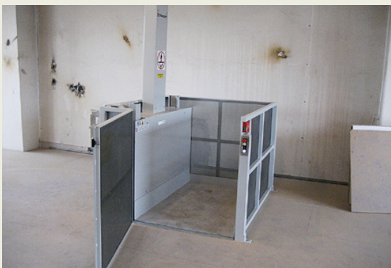
Quick and smooth installation.
