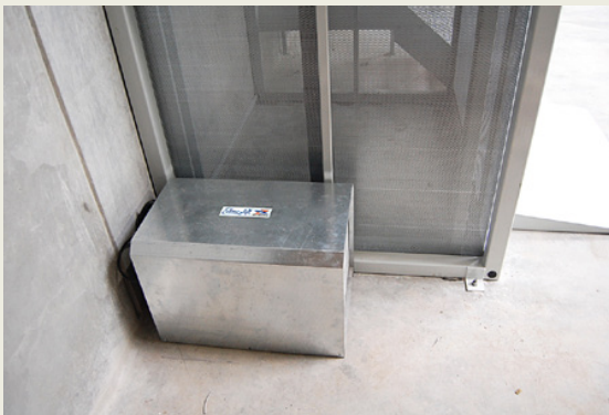
External lockable power pack means that a machine room is not needed.
